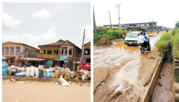
Figure 1.1: a) wastes dumped on road dividers; b) uncollected waste in the neighbourhood in Ijebu-Ode. b) silted drain with growing plants and its impact on roads in Ijebu-Ode (Aiyewunmi, 2023).
