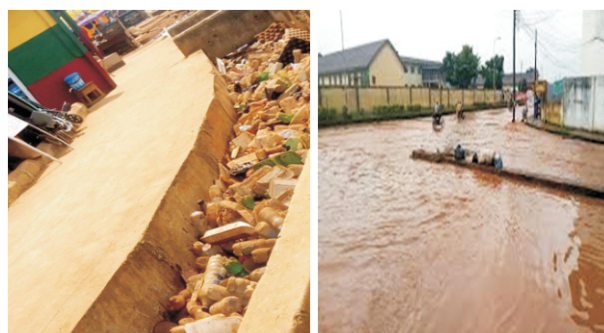
Figure 1.2: a) excessive rubbish in the drain in Ijebu-Ode; b) flooded streets/roads and narrow and blocked drainage in Ijebu-Ode (Aiyewunmi, 2023).
